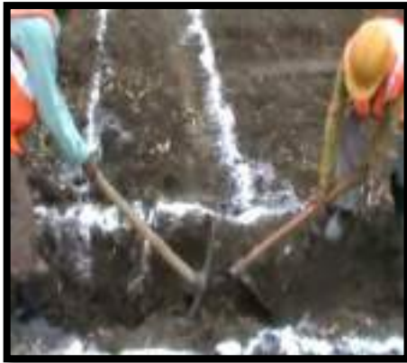
Cross Pit and Lime Powder Marking
